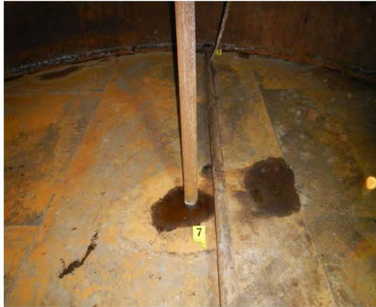
Figure 16. Retrofitted welded bottom of tank 396 (inside of tank). (Source: CSB)
