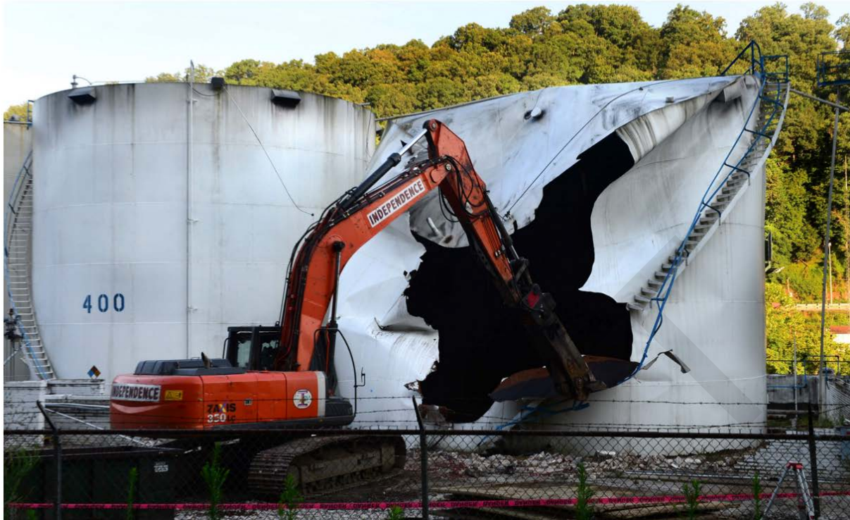
Figure 7. Demolition of the tanks at Freedom. 63 (Source: CSB)
