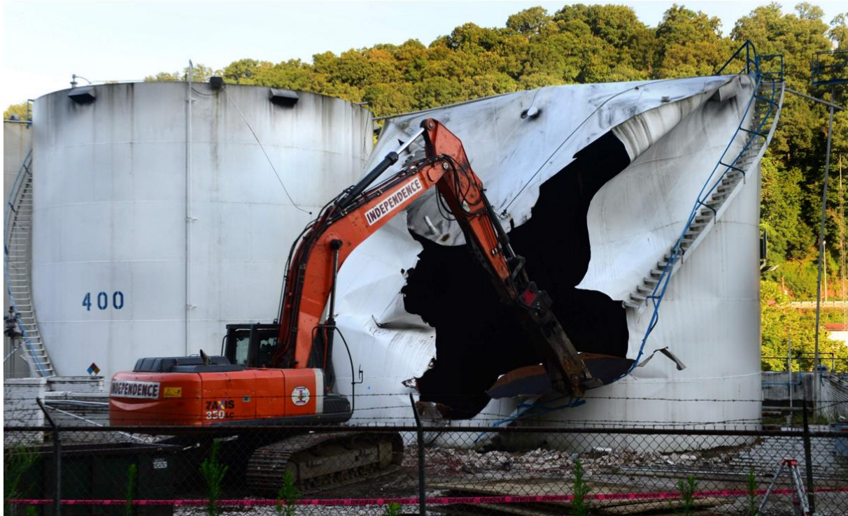
Figure 7. Demolition of the tanks at Freedom. (Source: Charleston Gazette)
