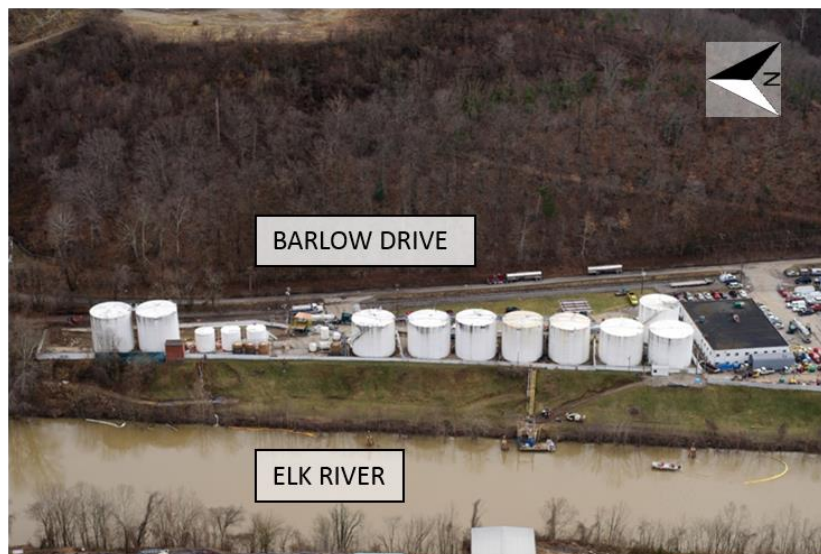
Figure 2. Etowah River Terminal located between Barlow Drive and the Elk River. (Source: CSB)
