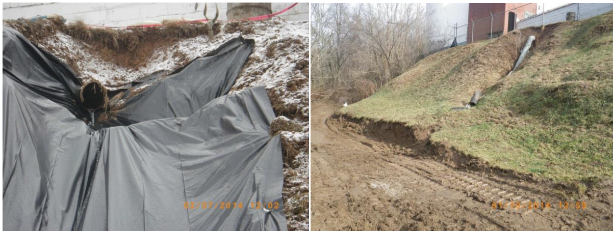
Figure 27. Water flowing through a corrugated steel culvert extending from the hillside (Left); stormwater pipe above interceptor trench (Right). (Source: WVDEP)
